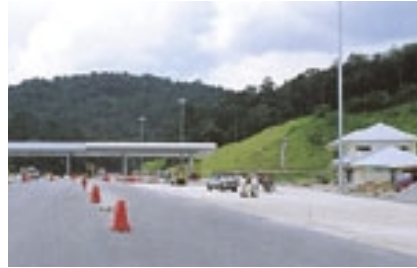
left: Toll plaza nearing completion at the East Portal of SPRINT's Penchala Link.
