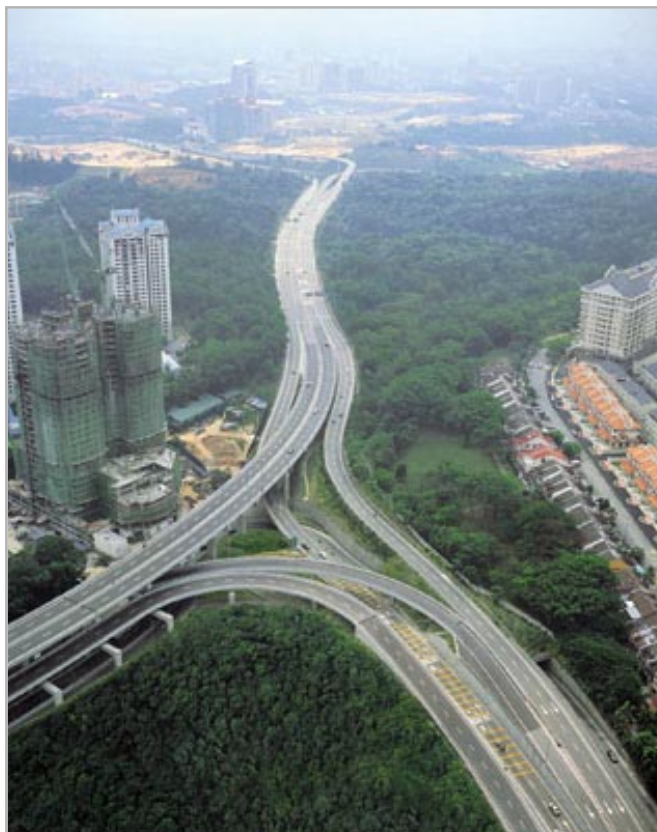
Mont Kiara Interchange on Sprint, is a 3-level, Y-interchange connecting Penchala Link and Kerinchi Link.
