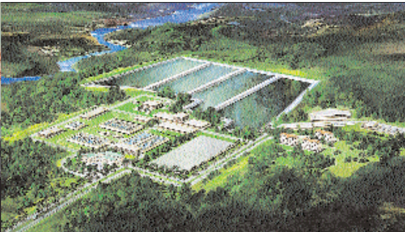
Rasa water treatment plant Loji rawatan air Rasa
