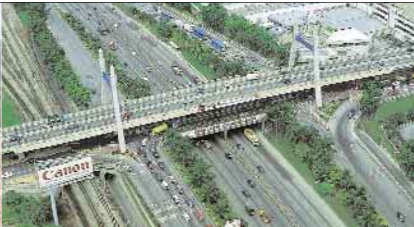
LDP Cable-Stayed Bridge Jambatan Tambat Berkabel LDP
