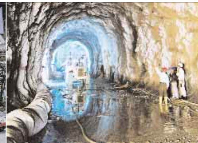
Diversion tunnel at SSP3 damsite Terowong lencongan di tapak empangan SSP3
