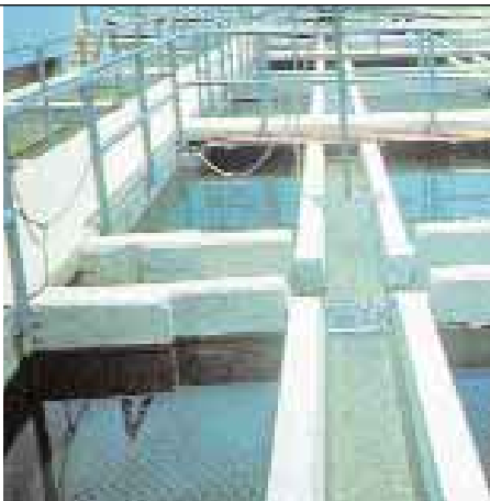
Sungai Selangor Water Supply Scheme Phase 1 (SSP1), sedimentation tanks and control room Skim Bekalan Air Sungai Selangor Fasa 1 (SSP1), tangki empangan dan bilik kawalan
