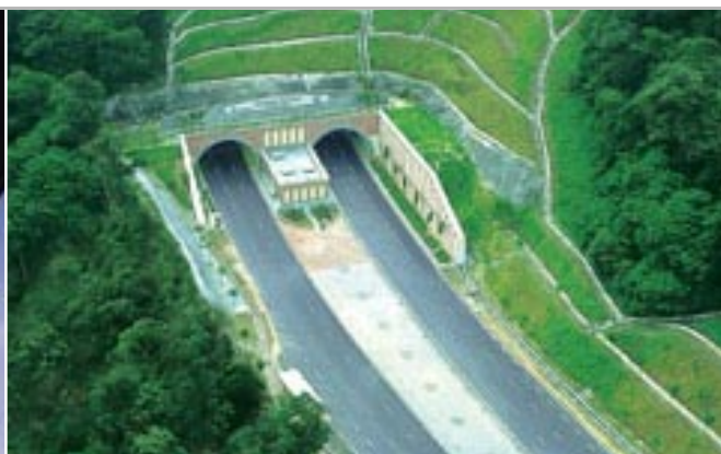
West Portal of the unique twin-tunnels of Penchala Link. Gerbang Barat terowong berkembar unik di Hubungan Penchala.
