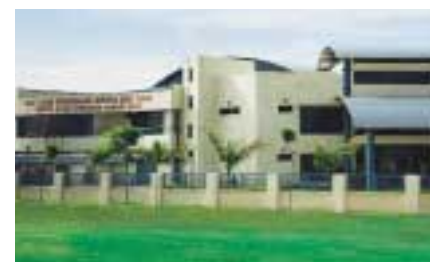
GPOS building at Kota Kemuning.
