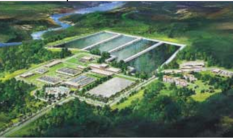
Rasa Treatment Plant.
