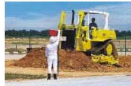
Plant operator operating on the excavator to hand signals.
