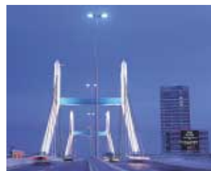
LDP Cable Bridge.
