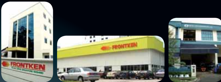
Frontken (Singapore) Pte Ltd - Jurong Plant 1 and 2, Metall-Treat Industries Pte Ltd
