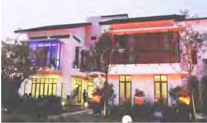
Glenmarie Gardens high-end villa development
