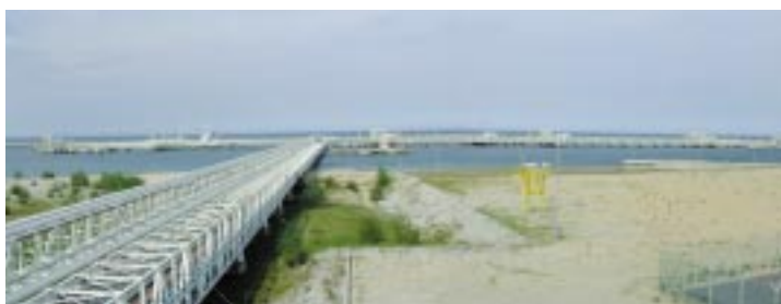
• Jetty main trestle and jetty facility.
