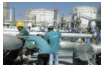
• Precommissioning work in progress.
