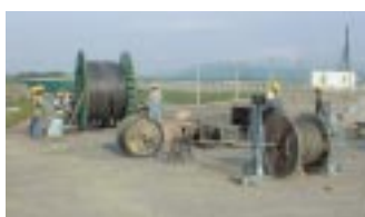
• 132kv cable laying work at south of Lot N.
