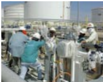
• Site installation of methanol mass flow metering skid.
