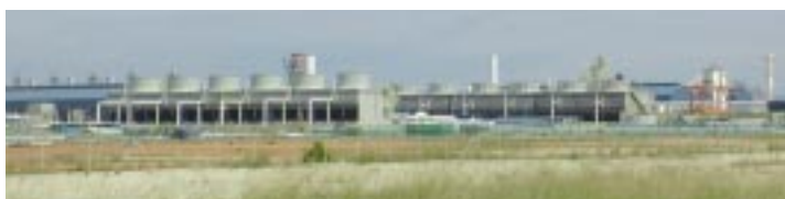
• General view of Petronas Gas Berhad Central Utilities Facility ("CUF"), Kertih.
