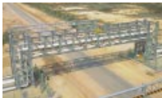
• Pipebridge at Gebeng.
