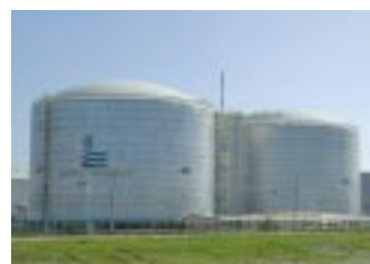
• Two nos. 45.0m diameter x 27.2m height refrigerated ammonia tanks.
