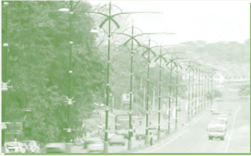
The Upgraded Jalan Tampoi
