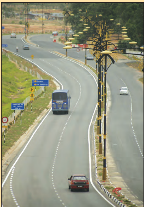
The upgraded Jalan Tampoi
