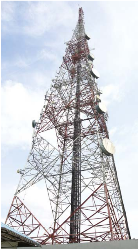
↑ SACOFA's Four-legged telecommunications tower
