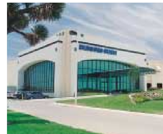
The new Dunham-Bush factory at Nuevo Leon, Apodaca, Mexico.
