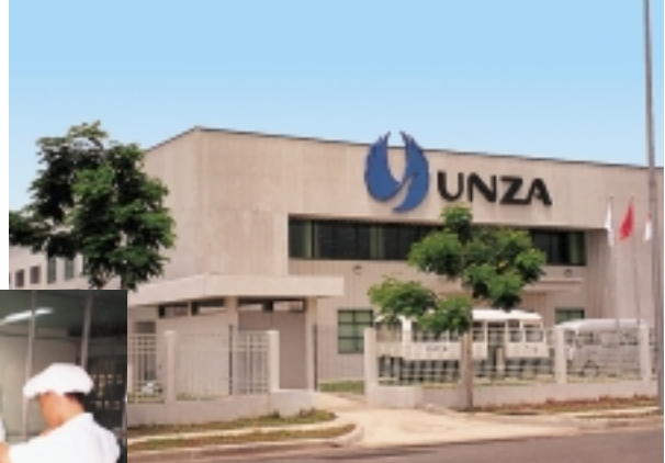
Unza Vietnam's factory in the Vietnam Singapore Industrial Park, the first outside Ho Chi Minh City.
