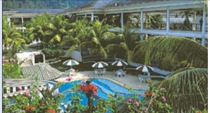
Kelab Darul Ehsan, Ampang, Malaysia - Pool View
