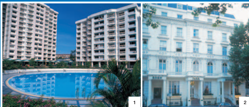
1 Petaling Indah Condominiums, Kuala Lumpur
