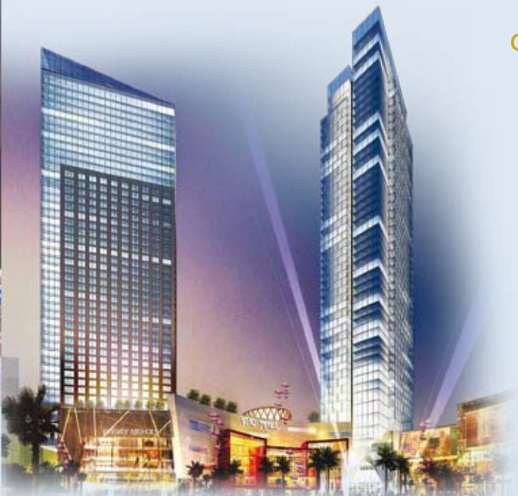
The proposed Vietnam Financial Centre, Ho Chi Minh City, Vietnam, is a mixed commercial development with offices, shopping malls, a 5-star hotel and service suites.
