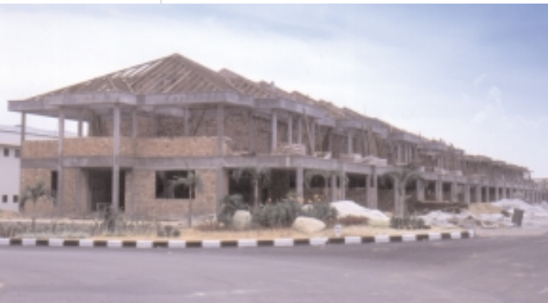
On-going construction, double storey terrace Phase 28, Taman Sri Kluang.
